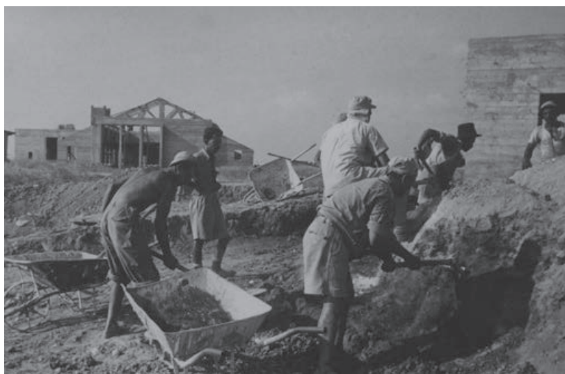
Fig. 1.10. Construction work at Ohalo, 1949 (courtesy, Kinneret archives).
