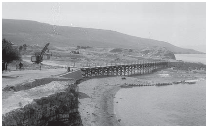
Fig. 1.5. Earth-quarrying by the Palestine Electric Company in April 1933.
