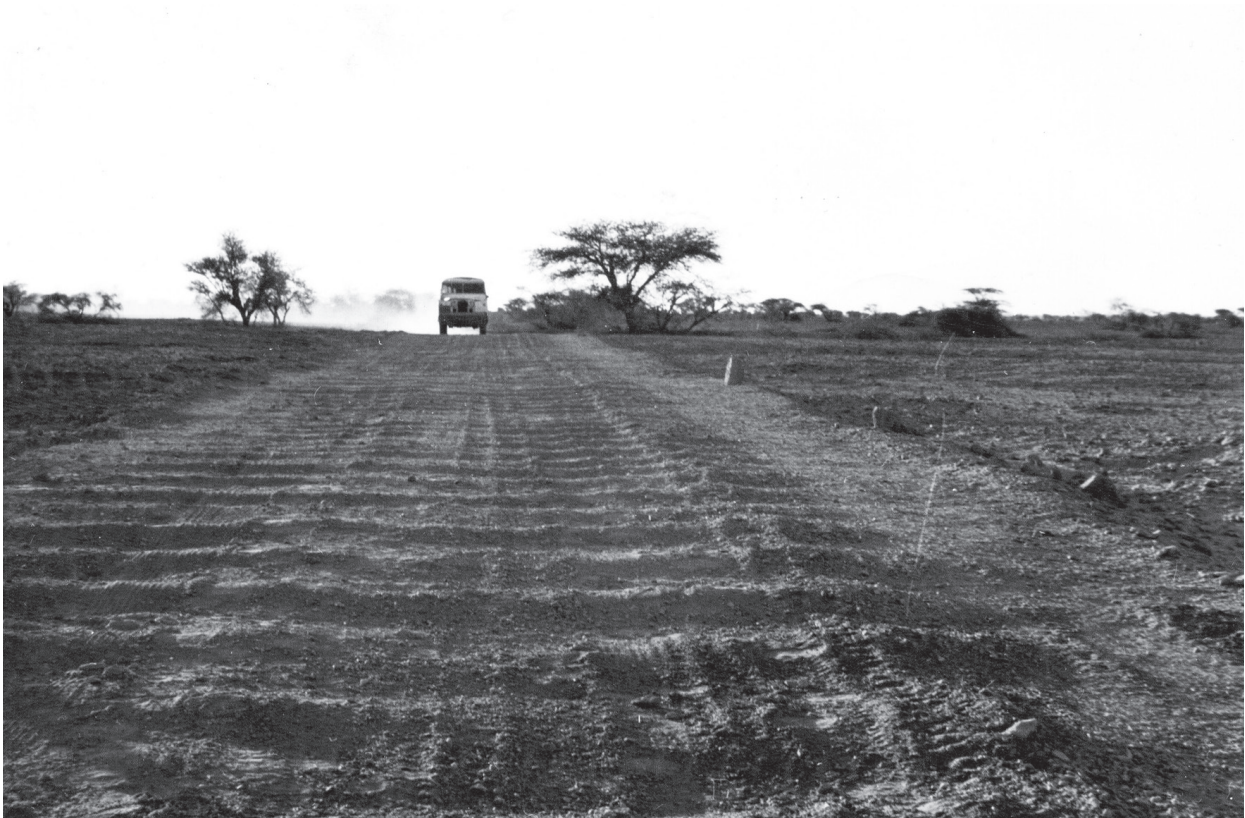
Figure 1.16. A famous peril of desert motoring in the pre-tarmac era – the washboard tracks (Philip Ward archive).
