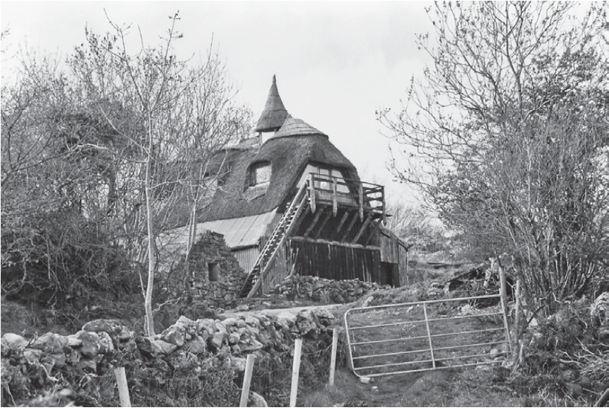
Figure 1.1 Fairy-tale turreted house, for a blow-in cheesemaker, County Clare, west Ireland.
